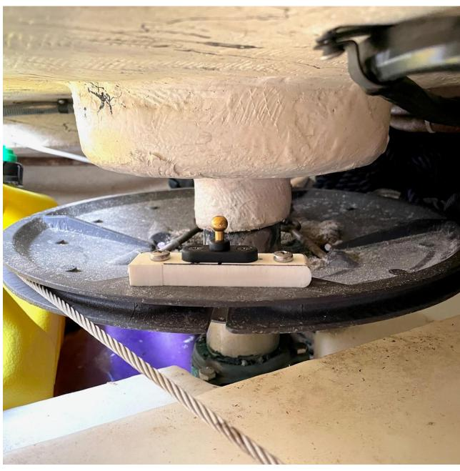
4. **Use Raymarine template to locate hole locations then pre drill for the mounting screws.** If you don't want to buy the right-angle drill, then you'll probably have to remove the water tank.
